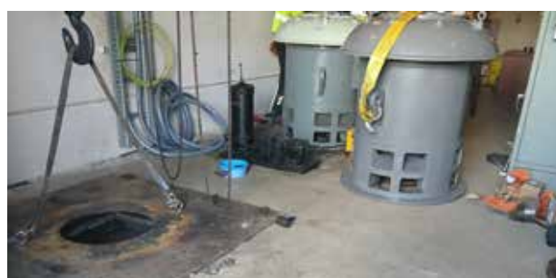
Installation works of reconditioned storm water pump 1 at Pump House 3, Drumgeely, Shannon.
