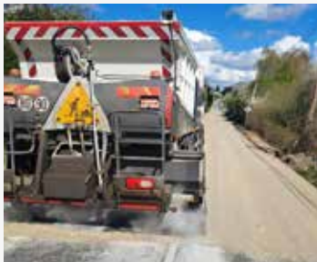
Sealing Clause 806 on the R-352 at Derrainy, Whitegate, Co.Clare
