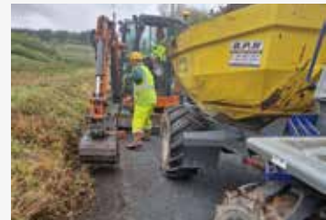
Road Prep for Surface Dressing on the L-8104 at Balloughtra, Tulla, Co. Clare
