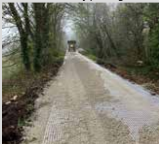
Laying of Secugrid on the L-8056 Golf Course road in Bodyke in advance of paving works
