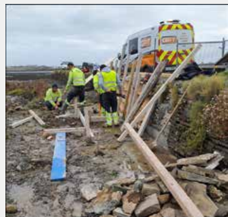
Repairs to Sea Wall defect.
