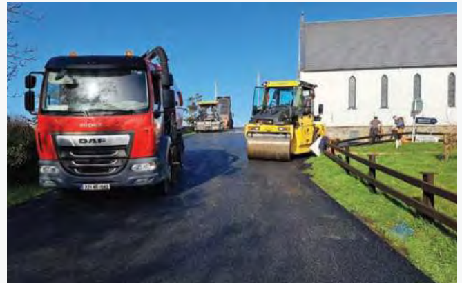
Overlay works on the R-479 in Doolin
