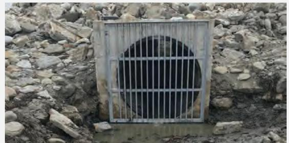
*Replace damaged pipe grids on 2 large surface water outfall pipes in Quilty*
