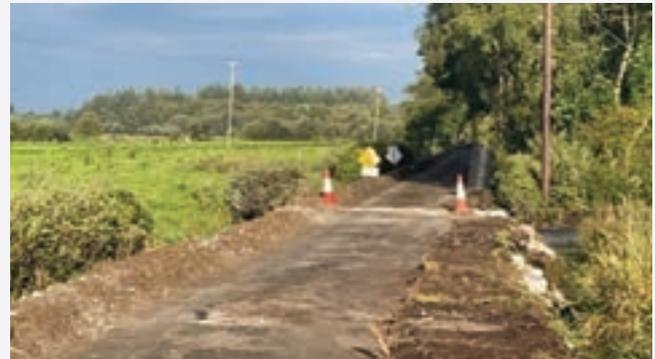
Works at CIS project at Errinagh. Road crew carrying out drainage and banking works.
