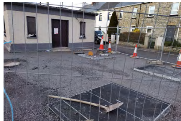
Clarecastle Quay Road
