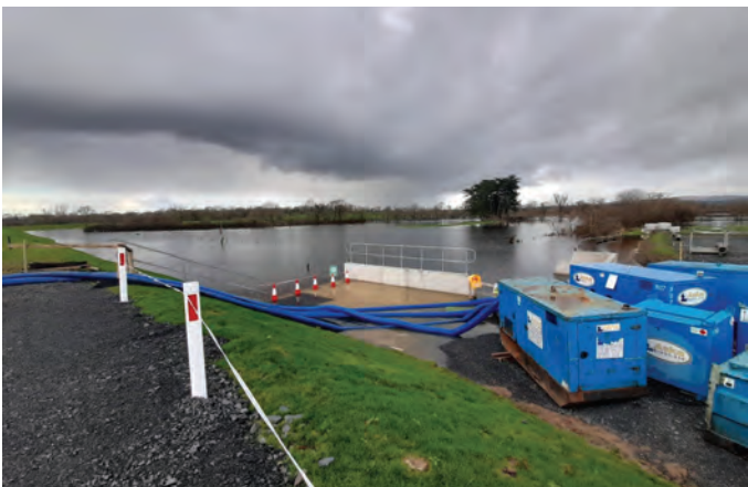
Pumping of flood waters at Embankment Works
