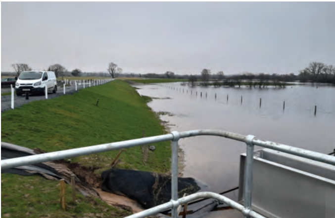
Shows the rising levels of water at Embankment Works in Clonlara.
