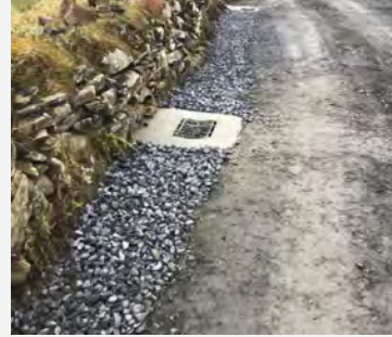
LIS Lissycasey, Installation of drainage
