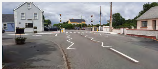
Ruan Village – pedestrian crossing and traffic calming works
