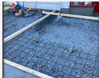
Doonbeg village, Improvements to footpaths to improve access for the mobility impaired.
