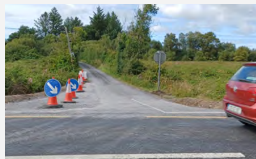
Tullycrine Junction improvement works.
