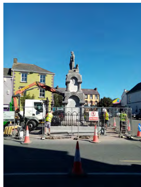
Installation of restored wrought-iron railings. Photo by Kilrush & District Historical Society.
