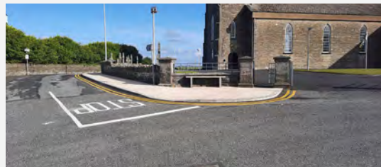
Milltown Malbay Church – new footpath and public lights connecting car park to Church
