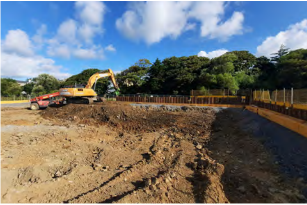
Kilrush cofferdam excavation
