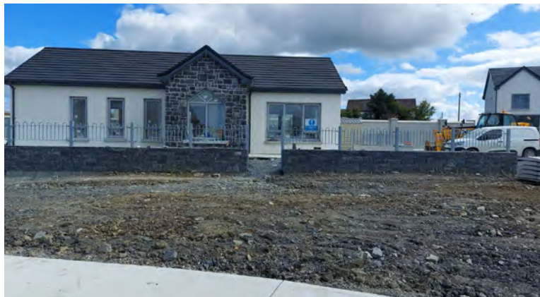
Miltown Malbay housing development which is due for completion later this year
