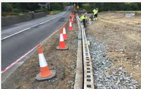
Ballynacally (R473, near GAA pitch), New footpath and wall.
