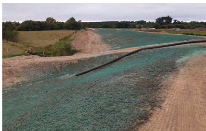
Springfield Embankment works
