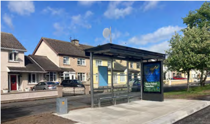
Newmarket on Fergus: Bus shelter.
