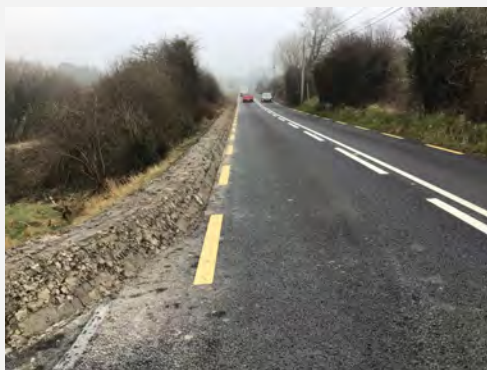
New earthen banking to recent pavement overlay - N68.
