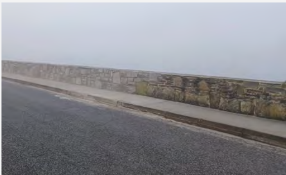
Replace stone cladding to wall - Cappa (Seán Crowley).
