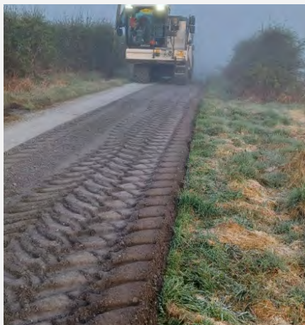
RR and Surface Dressing - Breaghwa.
