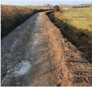
Road preparation works, Killernan.
