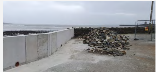
New RC Wall at Carrigaholt (old) Pier (ML Boland).
