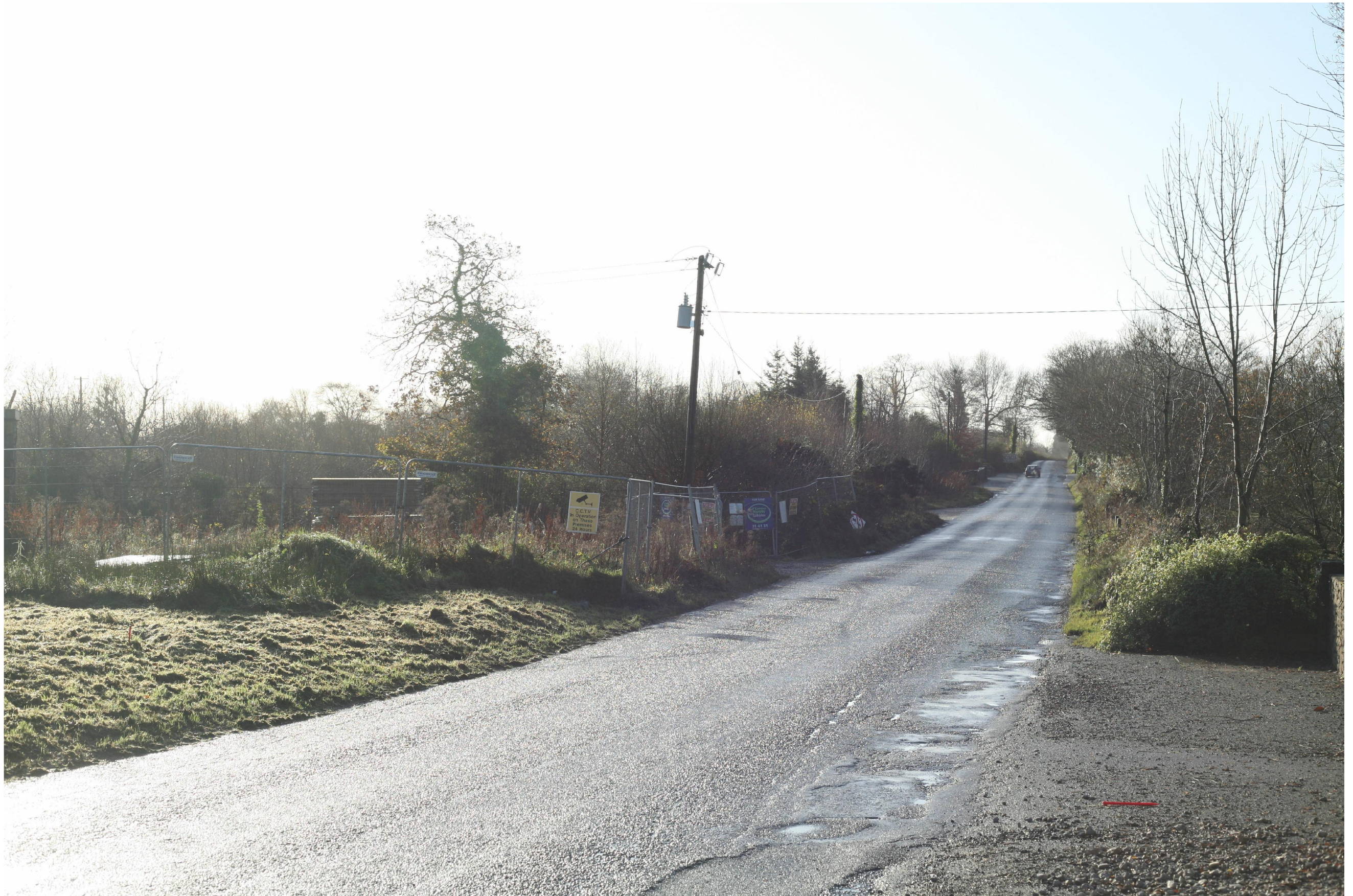
VIEW OF EXISTING R463 ROAD (LOOKING SOUTH) AT LOCATION OF PROPOSED INTERSECTION WITH SHANNON BRIDGE CROSSING/KILLALOE BYPASS
