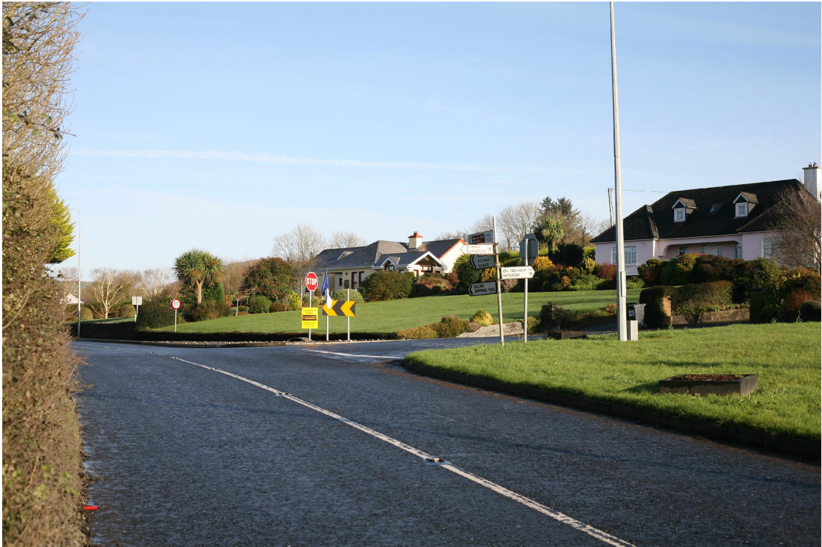
EXISTING VIEW OF R494 / R496 JUNCTION AT ROOLAGH (LOOKING NORTH)
