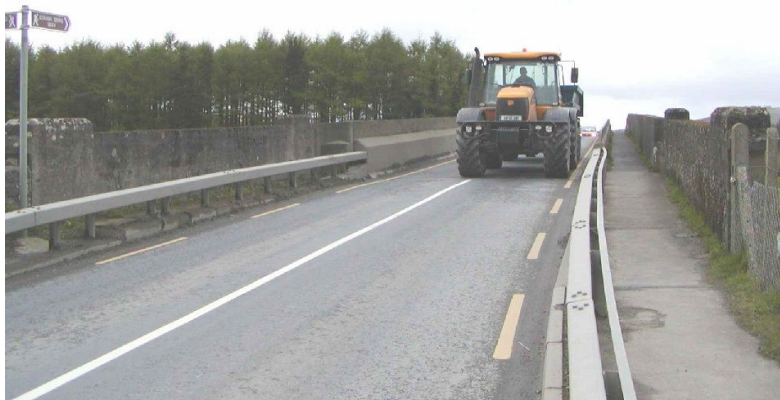
Figure 2.5: Headrace Canal Bridge
