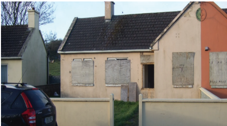
Vacant property before renovation
