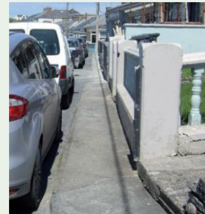
Inadequate Pedestrian Access
