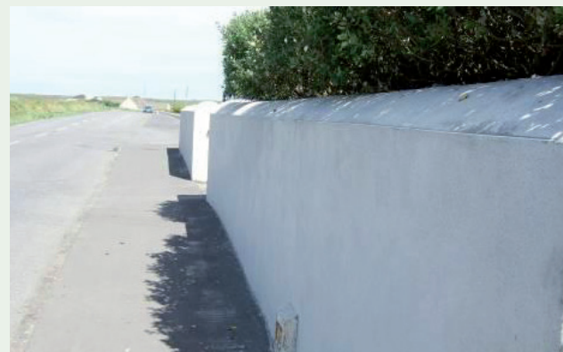
Uncapped Block Wall, Plastered and Painted
