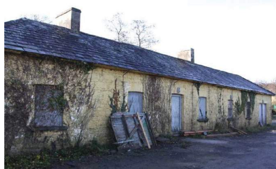
Former Steamboat Quay offices
