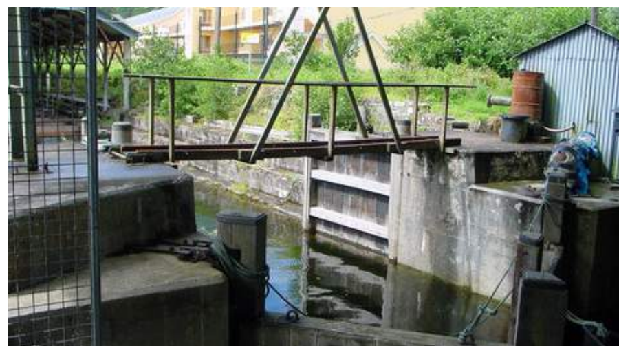
Inside the Dry Dock structure
