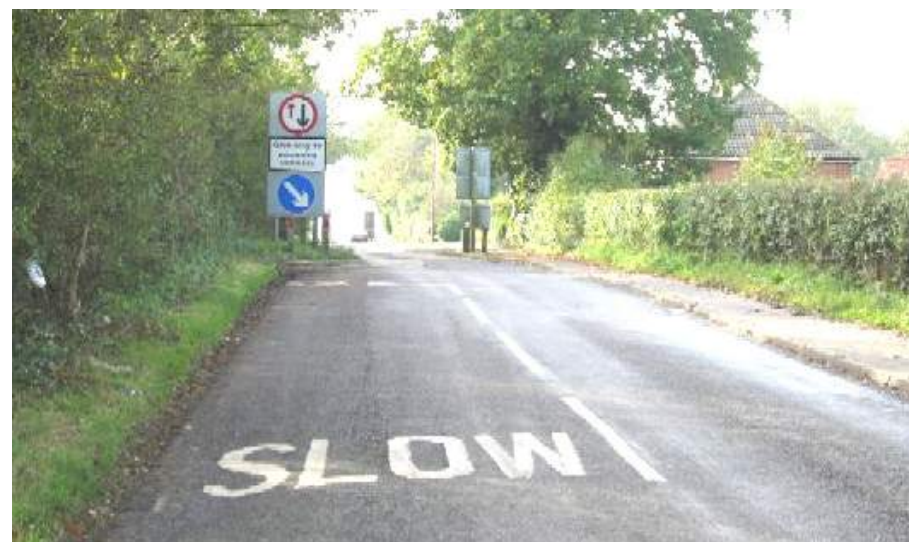
Typical 'Give way to oncoming traffic' and pinch-point measure as used in Britain
