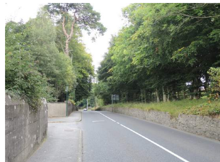
R463 on northern approach
