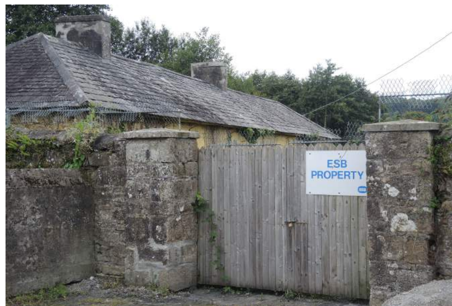
Existing entry to Steamboat Quay building
