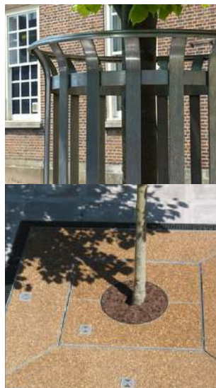
Typical tree guard and grille assembly
