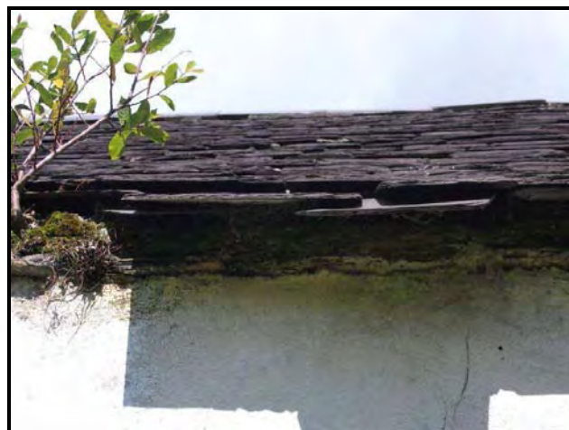
Image 3: Loose slates at edge of roof
