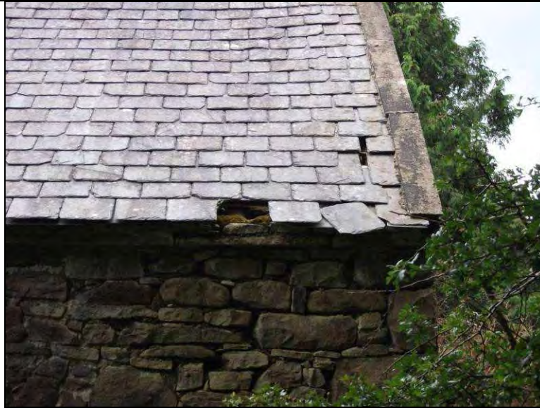
Image 2: Close-up of loose slates on roof
