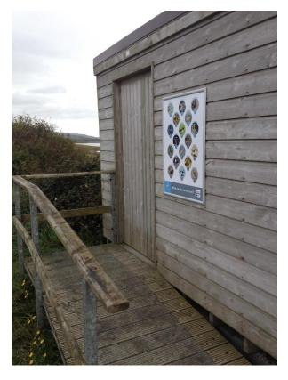
This hide (left)has its door placed sensibly on the rear and the access path runs behind the hide which in itself provide screening of the approach.
