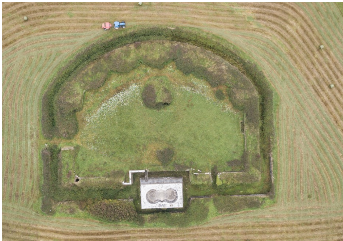
Aerial View of Kilkerin Battery Fort
