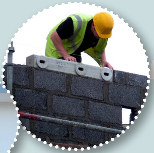
Swift boxes installed by tradesmen at build stage
