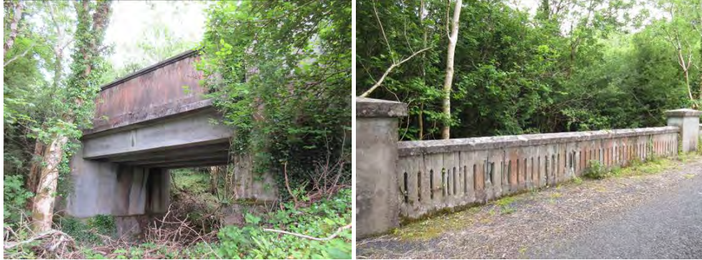
Fig. 35-36: Concrete bridge at Gortcurka (12) with concrete beam supports and precast balustrade
