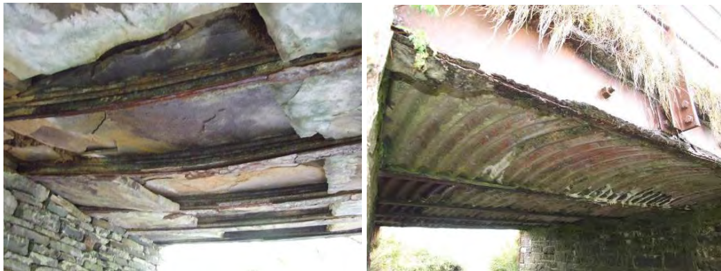
Fig. 12-13: Soffits of flag infill (7) and profiled metal infill (155)
