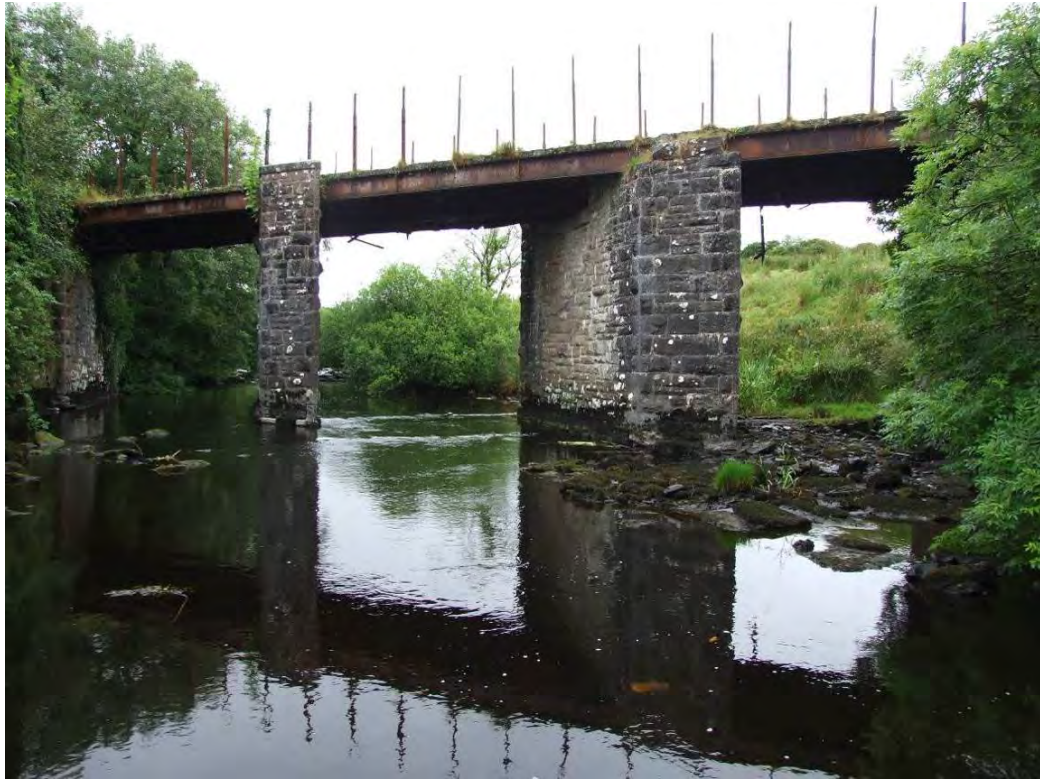
Fig. 32: Impressive former railway bridge (83) spanning River Inagh in Ennistimon at skewed angle and having skewed piers and abutments
