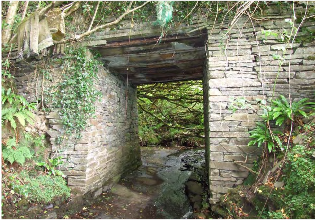
Fig. 4: Use of flat stones in abutments and soffit to bridge (65) at Silverhill/Glendine South
