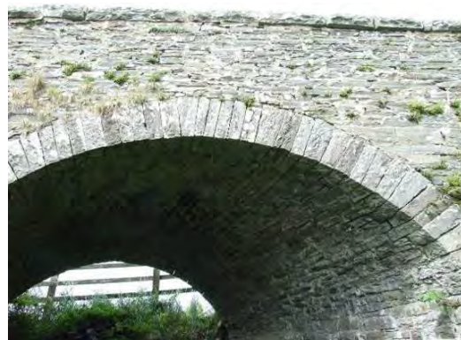
Fig. 33-34: Left: disused railway bridge over road (75) at Cullaragh South & Right: Road crossing a disused rail line at Fintra More (68), a stone bridge with a skewed barrel
