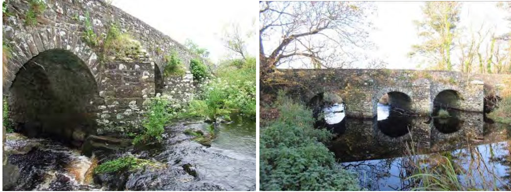
Fig. 6-7: Wide piers in bridges (Left: 107 & Right: 162) on the Aughyvackeen River suggesting early date
