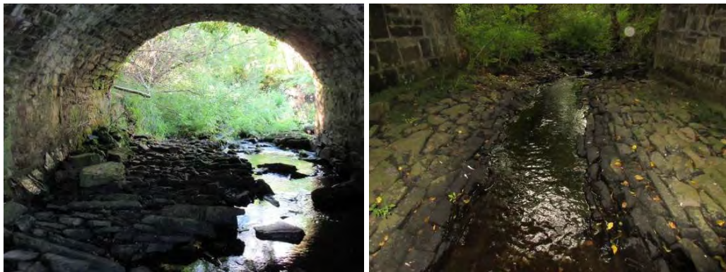
Fig. 8-9: Lapped bed stones at Inagh Bridge (24) and bonded pattern at Boola Bridge (20)
