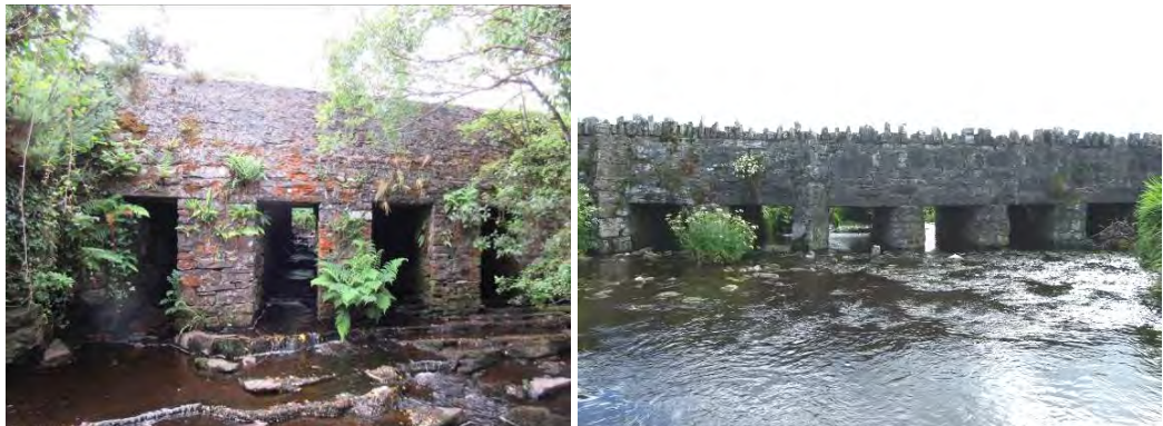
Fig. 5: Five-span Skagh Bridge (30) and twelve-span Doolin Bridge (97) using flat stones to span abutments
