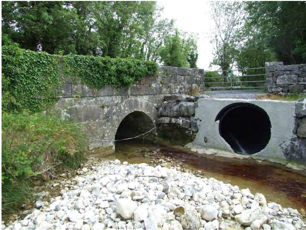
Fig. 43: Bridge at Drumbrickau (134): poor quality alterations adjacent to a fine stone bridge
