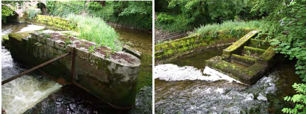
Fig. 10-11: Ashlar weir wall and mill race wall with two-span bridge (7)
