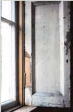
A cabinetmaker carried out some repairs to this shutter. The illustration shows new timber pieced in at the lower hinge, where decay had taken place, prior to repainting the timberwork
