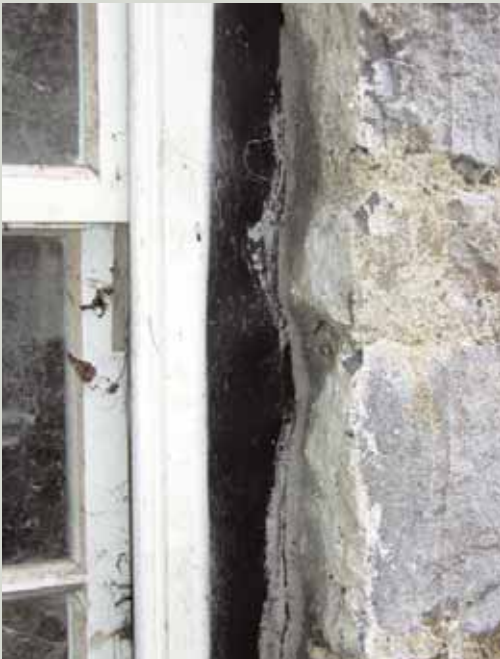
The silicone-based mastic used here is starting to lift in places, just a few years after being applied. As it is black and applied thickly it is more visible than caulking or pointing should be
