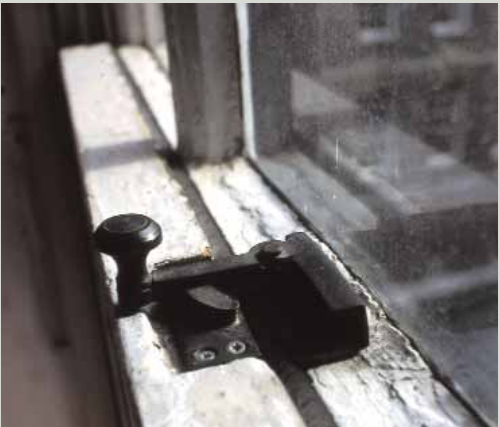
Draught strips come in several varieties. Brushes were fitted to this meeting rail gap. It is recommended that the advantages and drawbacks of each type are investigated so you know how effective they are likely to be. You should be assured that they will not damage timber joints and that catches and hinges can still function. Be aware of the approximate lifespan they are likely to have and be sure that they can be removed without damage to your historic windows
