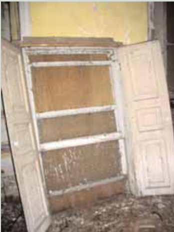
The window frame assemblage should not be removed from the structural opening unless this is necessary. If it must be removed, this should be done immediately prior to repairs being carried out, as otherwise the assemblage could be left vulnerable to damage
