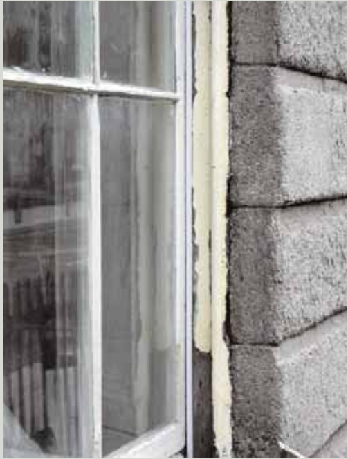
Many of the products require a patented plastic parting bead with inbuilt strips or seals to replace the timber bead. There is a visual impact from these proprietary fittings, especially those products only available in white, which limits the colours the window can be painted without drawing attention to them
