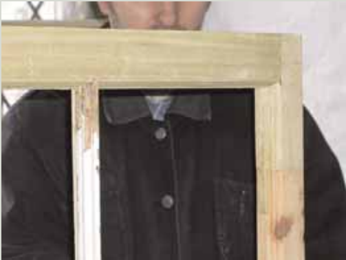
The cabinetmaker who made a new bottom rail and stile end (the sash is shown upside down) used a very strong mortice joint to fix the new stile end to the original. The moulding at the edge of the timber is accurate to the original
