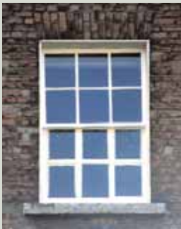
Over-cautious sealing of the putty by painting very far onto the glass can affect the appearance of the window, especially if it is not done consistently
