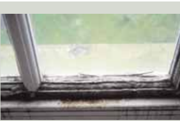
This mid eighteenth-century oak sash was dipped before being repaired with new parts. The ultimate effect of the chemical on the oak is obvious and serious: the original fabric is now incapable of repair
