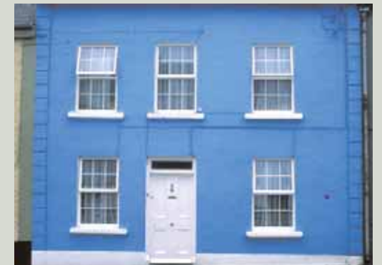
Possibly with the best of intentions, they were taken out and top-hung uPVC casements fitted instead. When closed these appear flat and insubstantial, and when swung open the superficial likeness to traditional windows is lost
