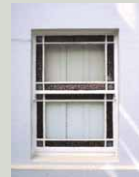
Some coloured glasses can be cut or etched to give a decorative pattern, as is the case with this window, which still has most of its original decorative margin panes with 'sunburst' corners
