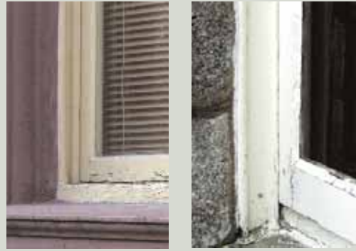
Generally, from the 1750s onwards the narrow sill seen here on the right became the standard, although the earlier 'full' (as shown on the left) sill remained common in Munster and was also used in imported nineteenth-century joinery
