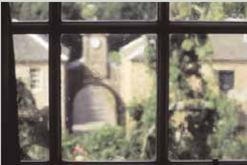
This film contains many bubbles and in general reduces the clarity of the view through the glass
