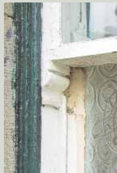
An early twentieth-century horn or joggle. The more slender the timber in a sash, the weaker the important joint at the meeting rail of the top sash, which bears all the weight of the sash as it hangs closed in position. Letting the 'horn' remain at this joint after construction, and decoratively shaping it, was a practical response to strengthen this vital joint. Generally, the smaller and plainer, the earlier the horn. More elongated and curvilinear shapes became common in the late nineteenth century
