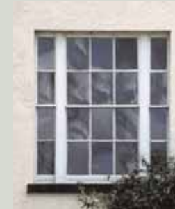
Historic glass types have a different appearance to modern float glass. They are wavy, often tinted or speckled and have a softer sheen. The presence of historic glass gives an irreplaceable visual quality to the appearance of an old window
