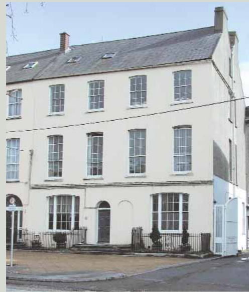
Elegantly arched windows are a characteristic of late Georgian Cork. The timberwork is also arched, an expensive option, but one taken by most original designers or owners
