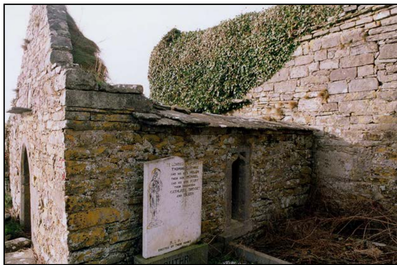
Figure 1: Kilmacrehy Church, Liscannor. View of 16 th century porch with stone slate capping
