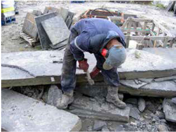
Despite machinery to lift, move and saw the stone, many traditional techniques are still used routinely.
