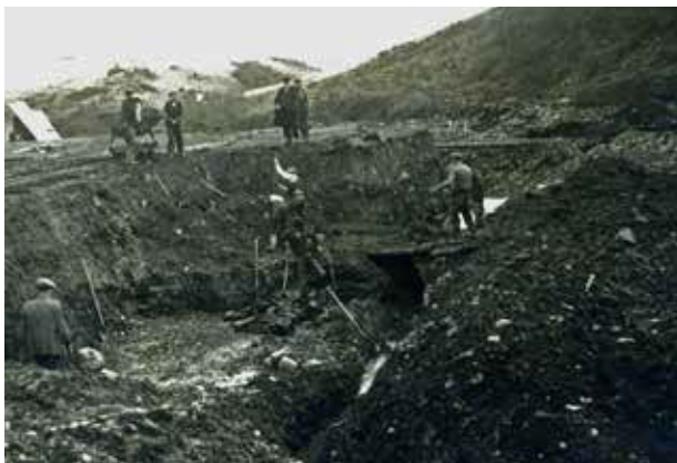
Toomullin: phosphate workings — bed near crusher, with about 8 foot depth of overburden
