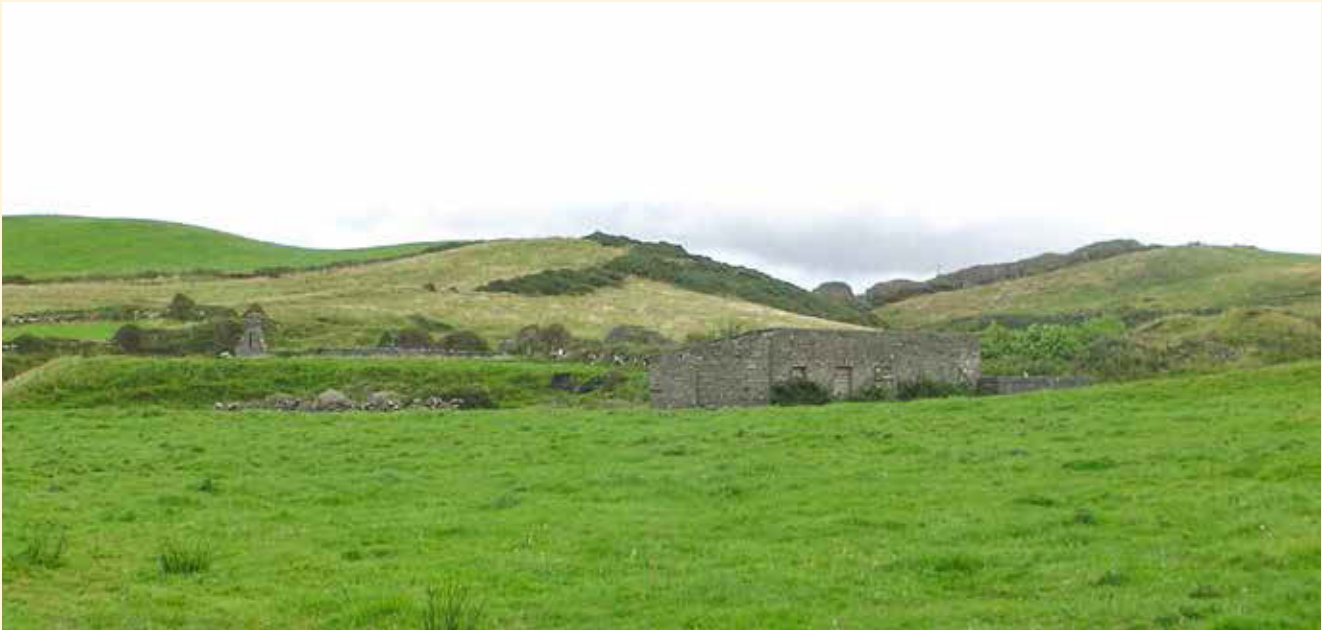
Small concrete building remains and spoil heaps can be seen from the road at Roadford.
