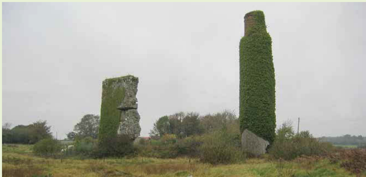
The chimney remains are cloaked in ivy, but only fragments of the steam engine house survive.
