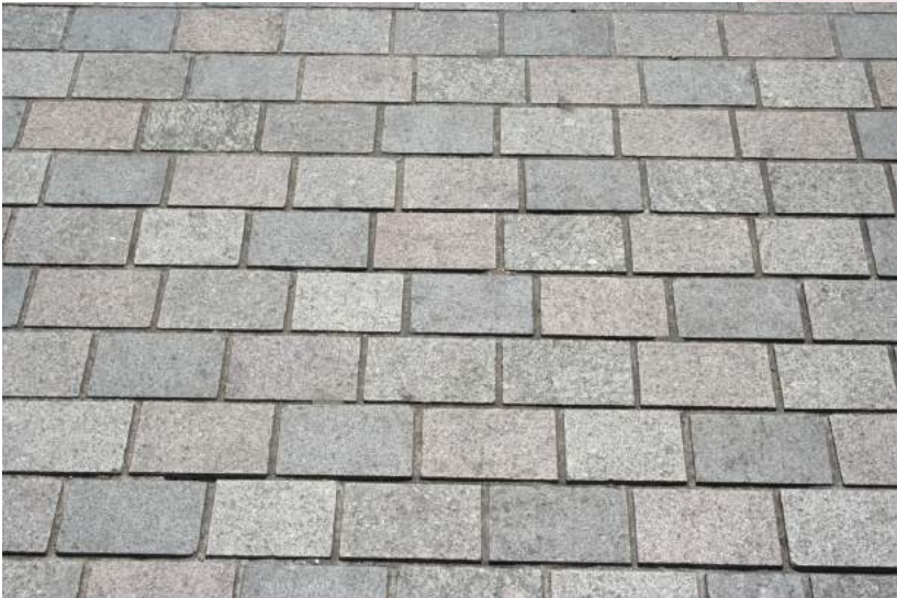
Re-surfacing: granite setts, multi-colour grey, 100x200x80mm thick, with Irish Limestone dished channel where required
