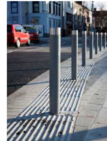
Corduroy tactile paving and bollards
