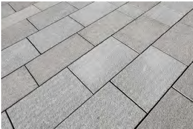
Paving Type 2: pedestrian-only areas Silver-grey granite slabs, staggered pattern
