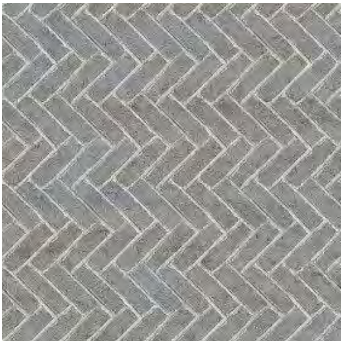
Paving Type 1: shared surfaces Multi-colour granite setts, herringbone pattern
