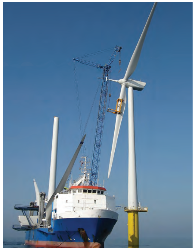
Photo 46: Construction of an offshore wind farm
