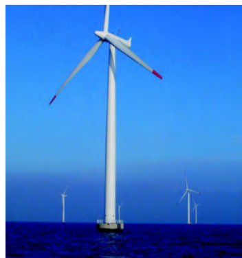
Photo 7 - Port Infrastructure is required to service offshore wind farms
