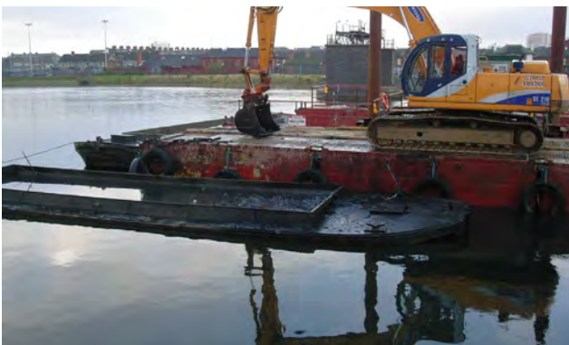
Photo 58 Dredging is an essential component of maintaining a safe and navigable waterway
