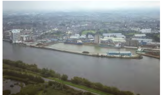
Photo 37 - Limerick Docks as a working Port
