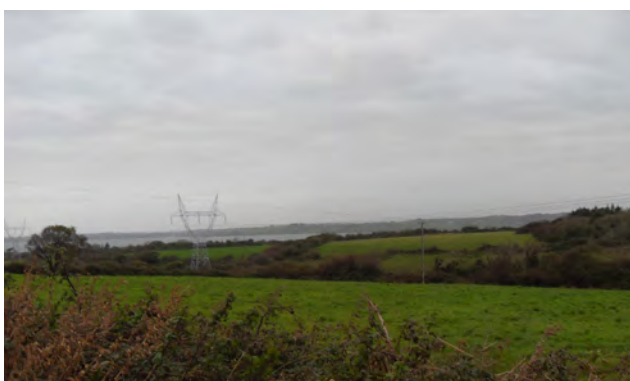
Photo 12 - Important grid infrastructure at Labasheeda
