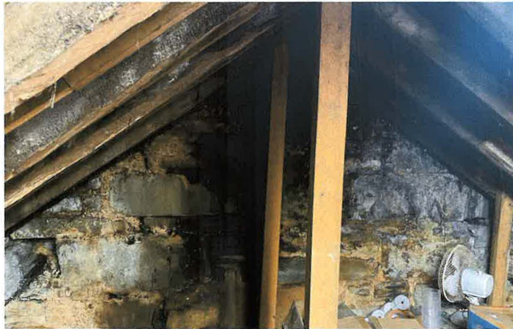
Damage to party wall from water ingress through chimney. Damage includes mortar washout, stone displacement and bulging to wall undermining the stability of the chimney structure
