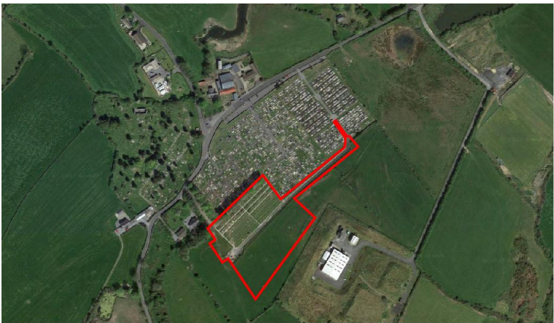
Figure 2.1.3 – Aerial Image of the proposed development site (image courtesy of Google Maps)
