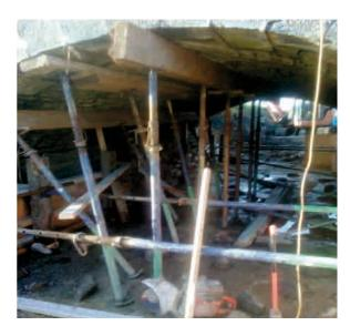
Clonbony Bridge N67 Miltown Malby: Emergency closure, river diversion, propping and repair due to flood scour damage.
