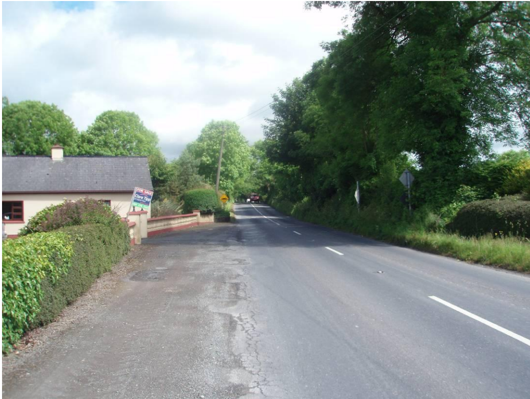
Plate 3.7 R494 approaches to Kilmastulla River Bridge looking northwards
