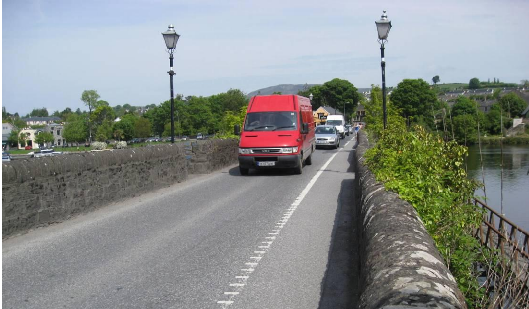
Plate 5.1 Killaloe Bridge with delineated pedestrian walkway
