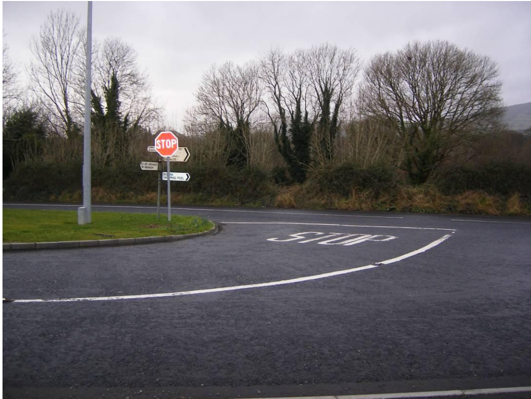
Plate 3.6 Roolagh Junction tie-in point looking east towards proposed Shannon Bridge Crossing
