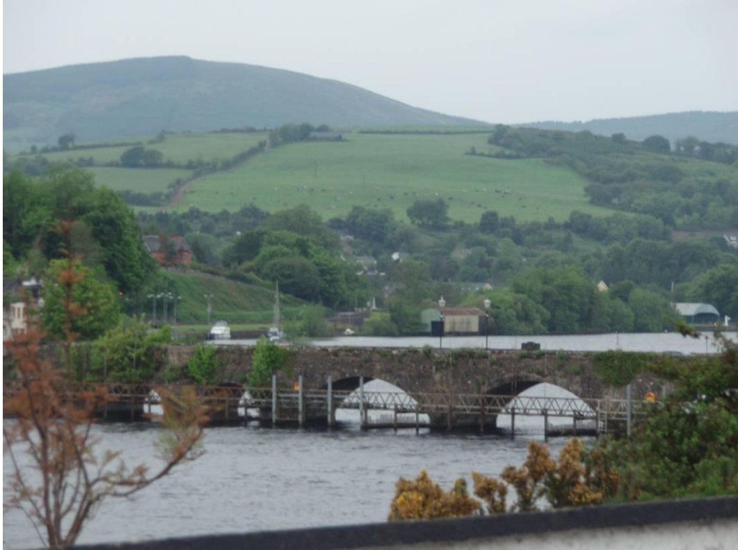
Plate 2.1 Existing Killaloe Bridge
