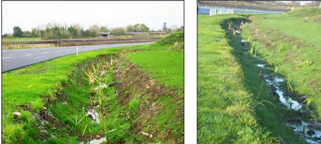
Plate 1.6 & 1.7 – Typical Planted Open Ditches (Over the Edge Drainage)
