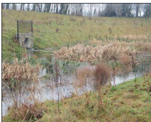
Plates 1.1 & 1.2 – Typical Constructed Wetlands/Attenuation Ponds
