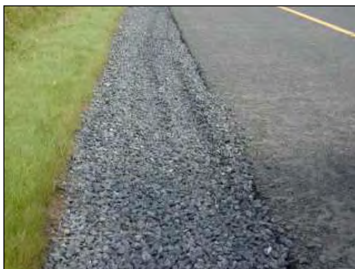
Plate 1.4 – Typical Filter Drain
