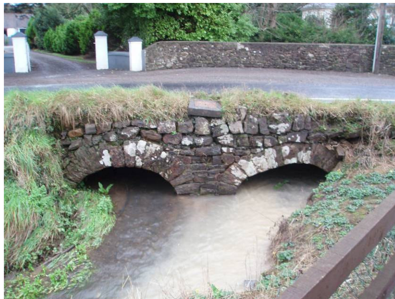
Photo 4.2: Unnamed watercourse adjacent to the R494 and N7 intersection (Doolly's Bridge)
