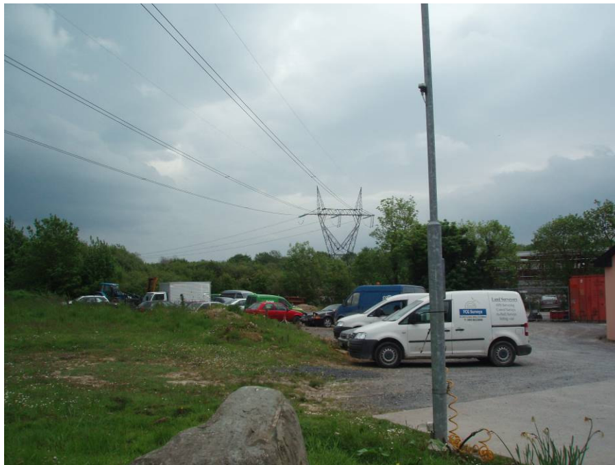
Photo 4.5 400kV transmission line crossing the R494 to the rear of the Esso Station
