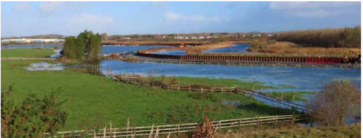
Sheet pile flood defence wall construction along the River Fergus.
