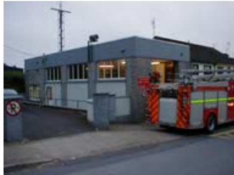
Killaloe Fire Station
