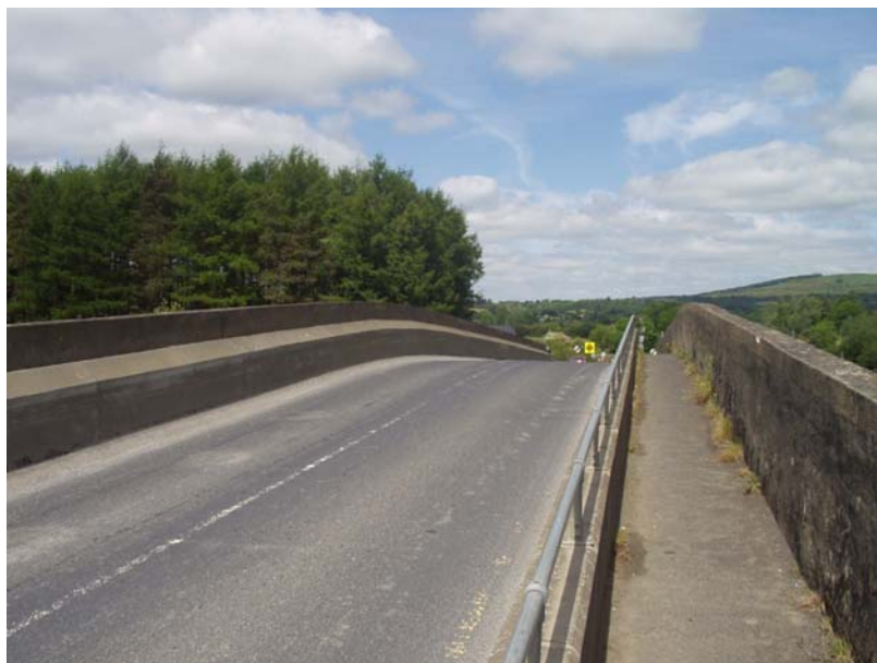
Headrace Bridge at O'Briensbridge
