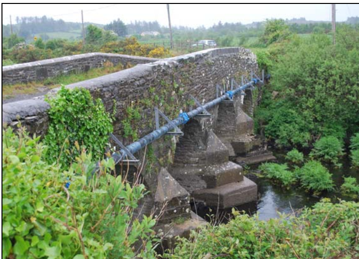
Plate 4: Moananagh Bridge, Co. Clare illustrating 'stepped cutwaters'
