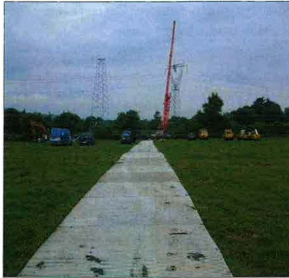
Figure 14: Temporary Aluminium Panel Tracks
