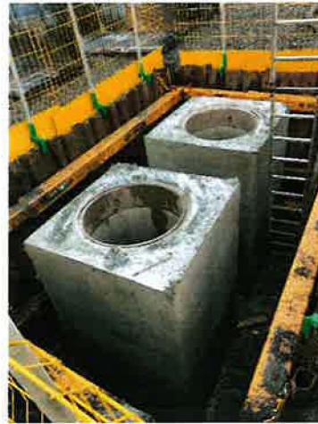
Figure 12: Raft foundation in poor ground conditions
