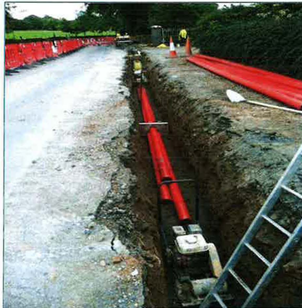
Figure 6: Typical 38kV Underground Duct Installation
