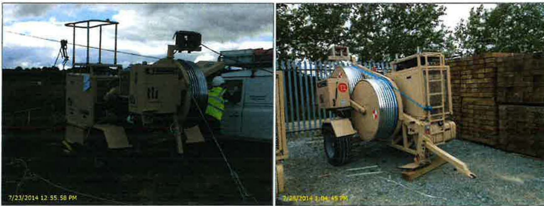
Figure 13: Puller – Tensioner Machine
