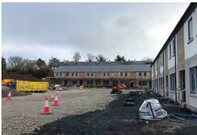
Works ongoing on Sixmilebridge project
