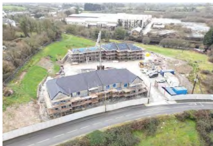
Progress on Scarriff housing development
