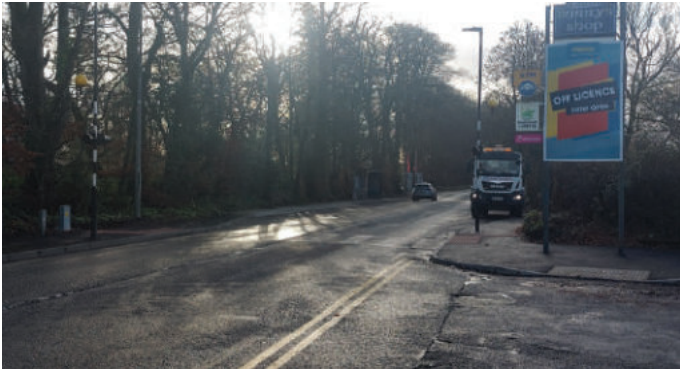
Pedestrian crossing and footpath upgrade at Barrys Cross, Ardnacrusha
