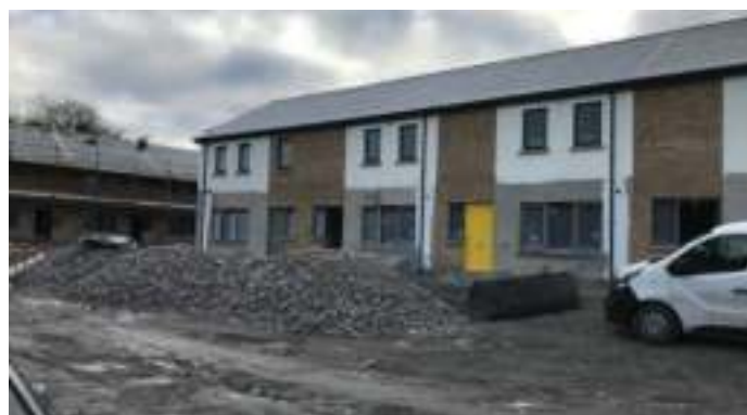
Works ongoing on Sixmilebridge project.
