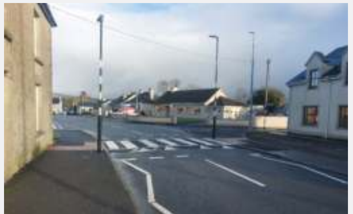
Completion of raised pedestrian crossing and junction tightening in Sixmilebridge
