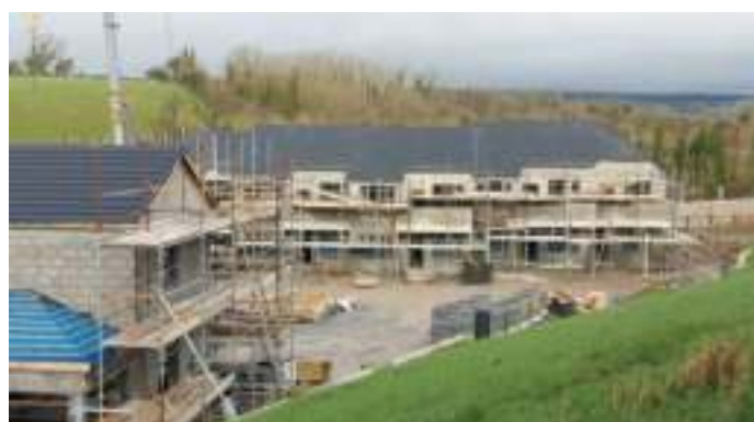
Progress on Scarriff housing development.
