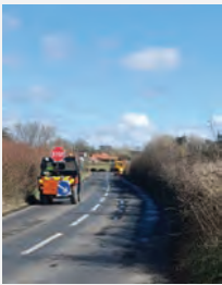
Drainage prior to road strengthening & resurfacing works in Cloonakilla,
