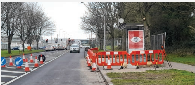
New bus shelter and associated works, Aidan Park, Shannon.
