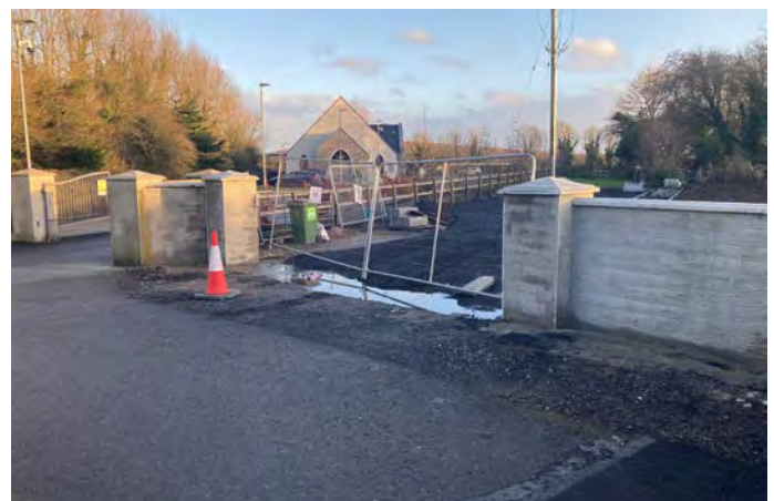
Site works underway at Hastings Farmhouse to improve accessibility.
