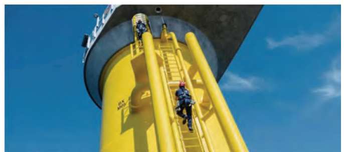
Wind turbine generator boarding ladder will be replicated on the quay wall
