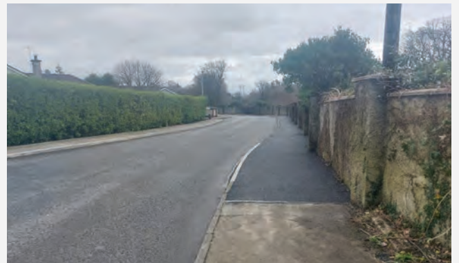
Footpath improvement works at Keelgrove, Ardnacrusha have been carried out.
