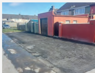
Foyle Park footpath improvement works.
