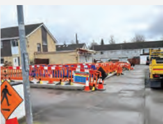
Works at Aidan Park.
