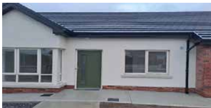
Completed bungalow at Hogan’s Place, Limerick Road, Ennis.
