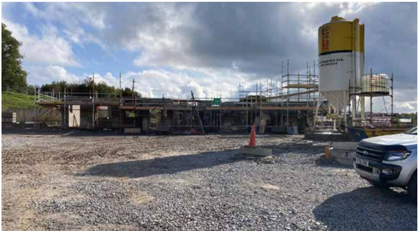
Progress on Scarriff housing development.
