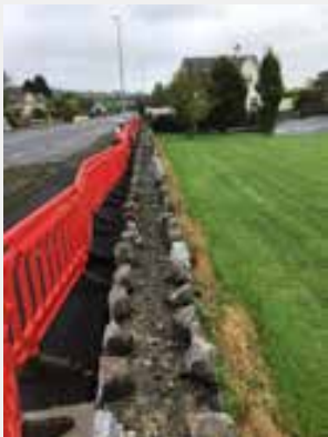
Footpaths & drainage works in Lissycasey
