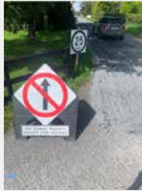
Surface Dressing at Ballyea
