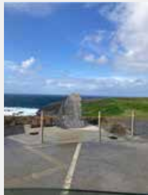
Memorial Plaque works at Kilkee Cliffs
