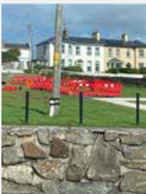
Pedestrian area works. East End, Kilkee
