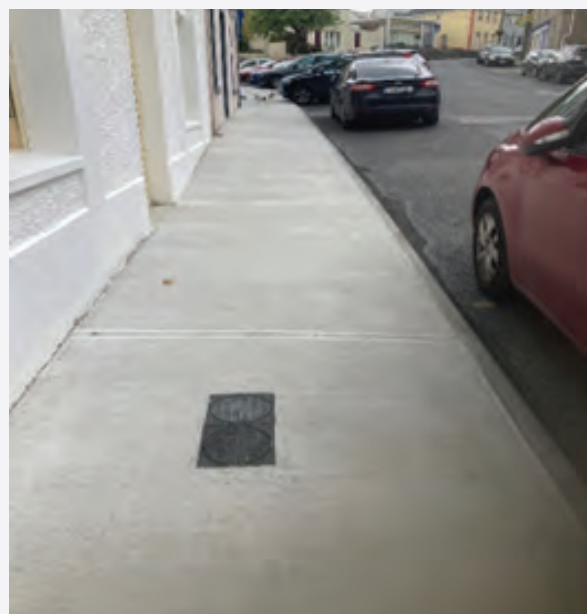
Completed footpath upgrade at Tulla
