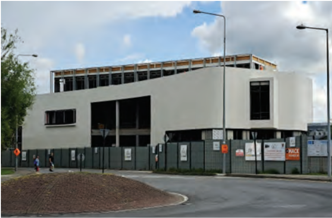
Current view of new County Library Project under construction.
