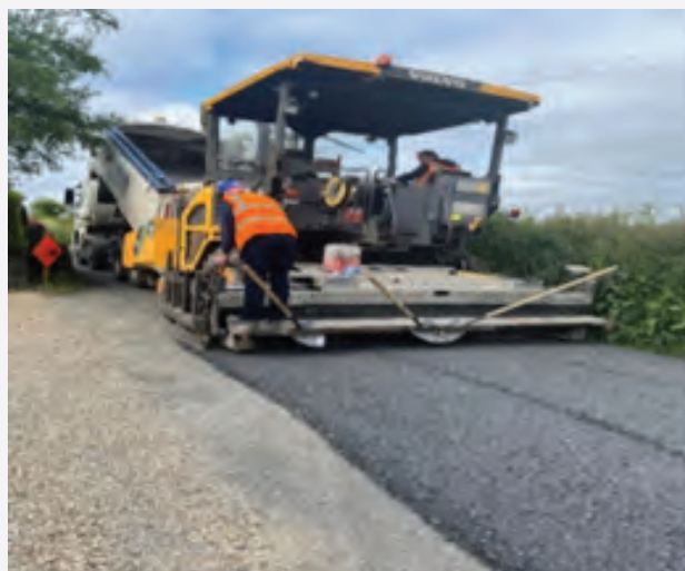
Surface Dressing Programme in progress
