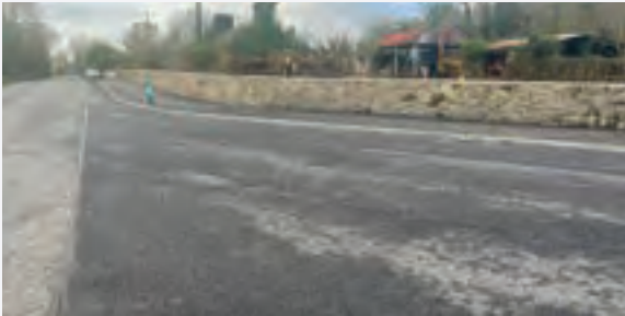
Footpath repair works at Nilands Service Station, Tuamgraney
