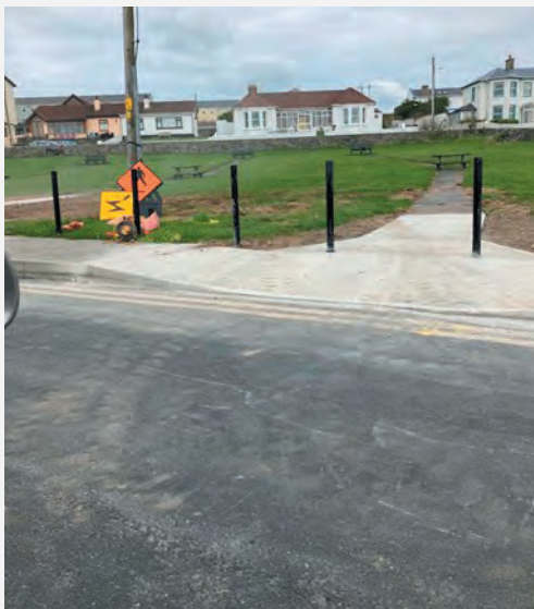
Works to improve footpath access for the mobility impaired in Kilkee.
