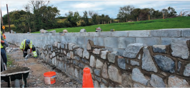
Works on the provision of a footpath in Ballynacally village.
