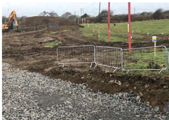
Kilrush WWTP site 28th Jan. 2022.
