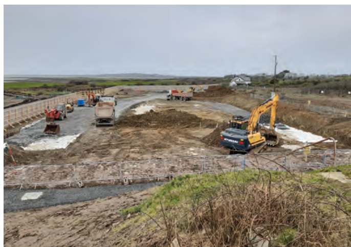
Kilrush WWTP site 17th Feb. 2022.
