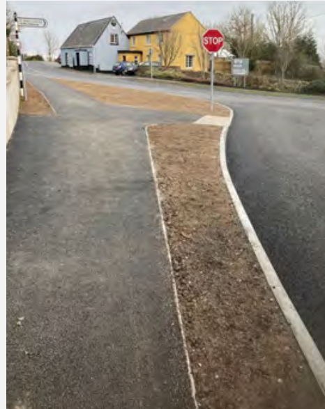
Kilmurry Village works
