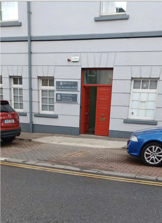
Drop kerbs at entrance to Kilrush Town Hall
