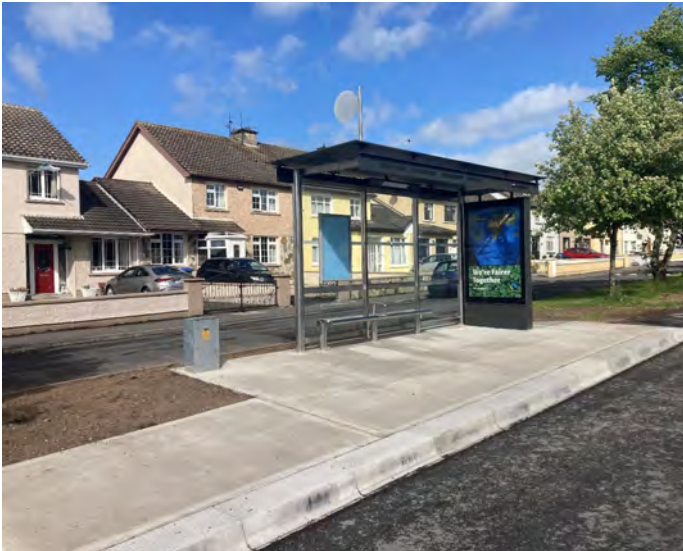
Newmarket on Fergus: Bus shelter.
